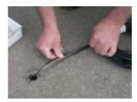
Cut a 5mm slot in tarmacadam road surface for the cable. Cut a trench for a duct in gravel or hardcore. Lower in the sensor until the yellow top is 8" below surface. Pour kiln dried sand in to fill the hole up to the top of the sensor. Fill the last 8" with a more structural plug of post mix or cold black top.
